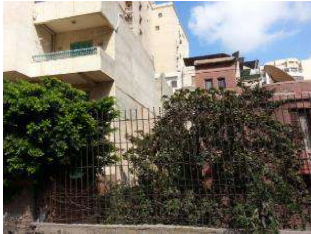
Figure 4-52: Newly constructed buildings
