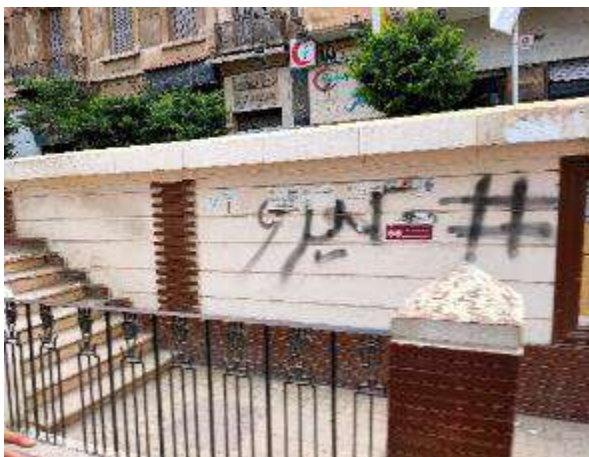
Figure 4-82: Concrete constructed fence
