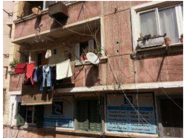
Figure 4-55: Buildings close to the tram fence
