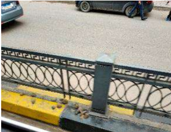
Figure 4-80: Fence close to Raml station
