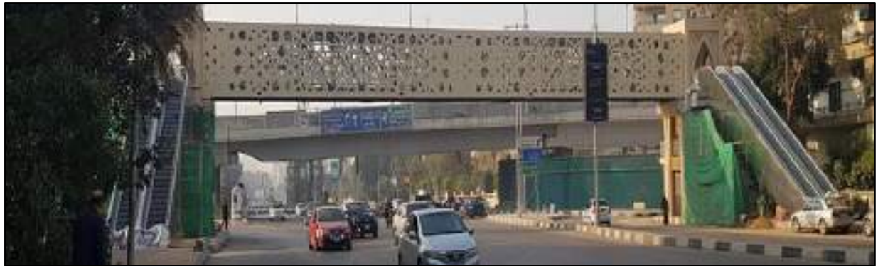
Figure 2-3 Example of Pedestrian Crossings
