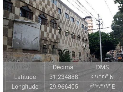
Figure 4-12: The mosque from outside (first mosque)
