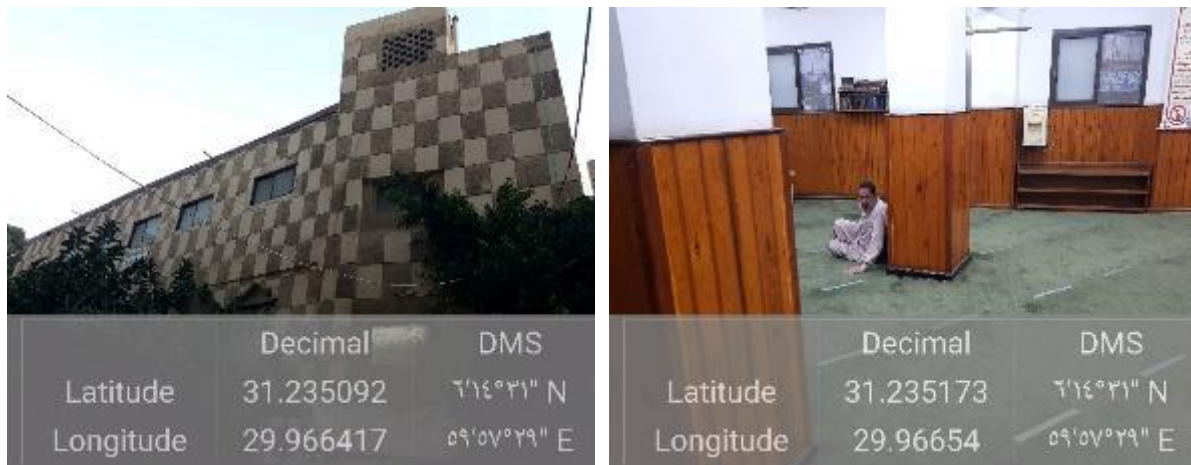
Figure 3-29: Mosque in Bakous station
